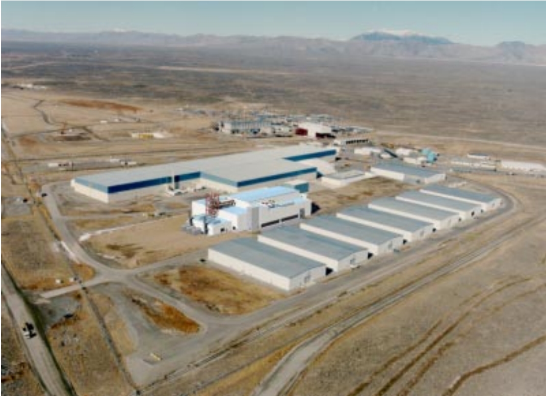
The artist's concept at left shows the new Advanced Mixed Waste Treatment Facility, center of photo, that is now under construction.
