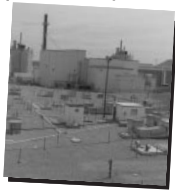
High-level waste stored in underground storage tanks at the Idaho Nuclear Technology and Engineering Center must be treated by 2035 and ready for shipment out of the state.
