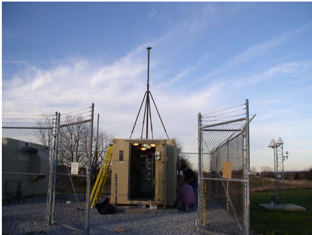
Figure 22. Photo of the Hagerstown GWEN site. In the back is the HAG2 site. On top of the hut is a pentapod with a marine antenna placed 4-5 meters above the hut in the search for cleanest signals. The HAG1 site was behind the camera. The 299 foot mast is several hundred feet to the right.
