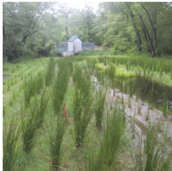
In June 2002, Peconic River pilot-study project shows great promise following sediment removal in March and replanting in April
