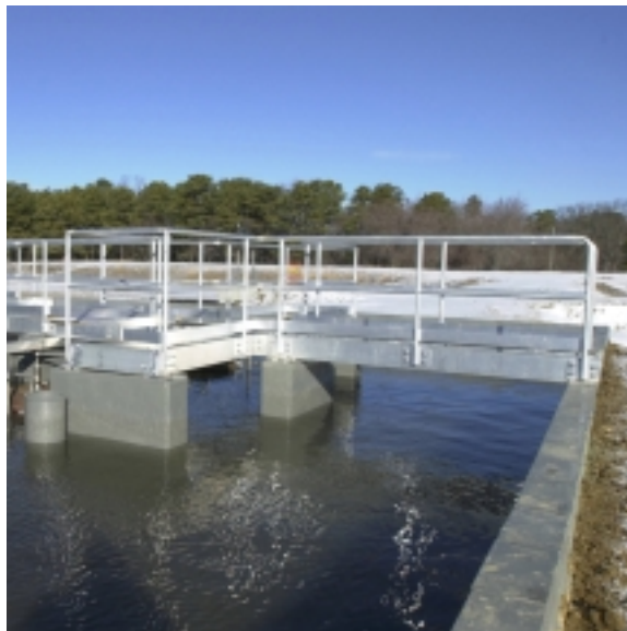
New Dosing Chamber at Sewage Treatment Plant (Sanitary Modification Phase II)
