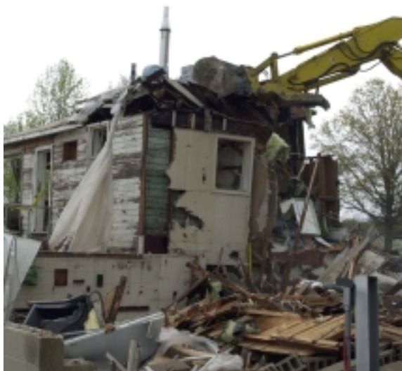
Building 318 being demolished
