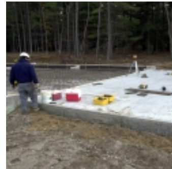
Newly poured rollup door apron for radioactive storage Bldg. 974
