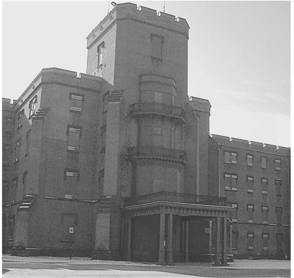
Figure 4: The Vacant Center Building, St. Elizabeths Hospital, District of Columbia
