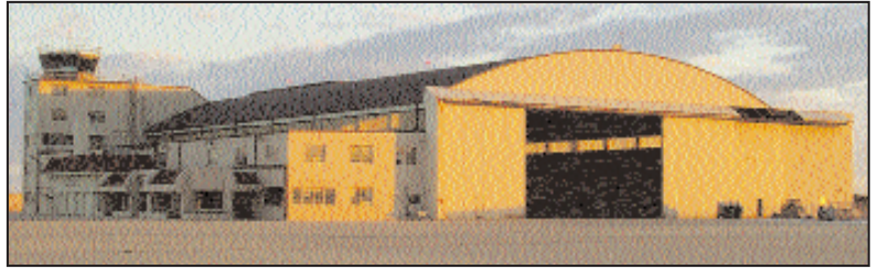
Hangar 800 is being demolished after 57 years of service as the base's main air terminal. It was replaced over the summer by a new terminal, supply warehouse and administration building. (Photo by Jim Laviska)
