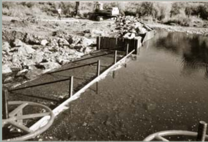
Lay-flat stanchion dam
