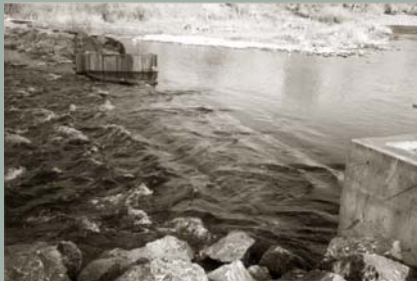
During the irrigation off-season, the dam's upright components are laid completely flat.
