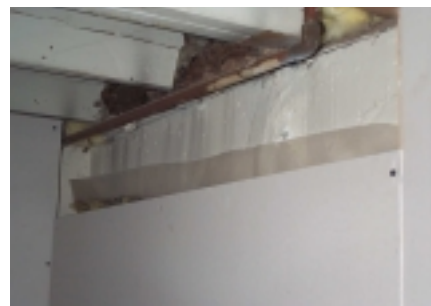
Basement rehab showing polyethylene behind drywall and framing.
