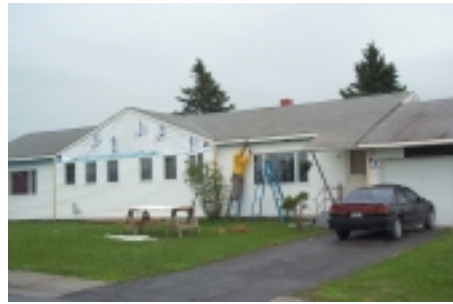
Installation of new siding.
