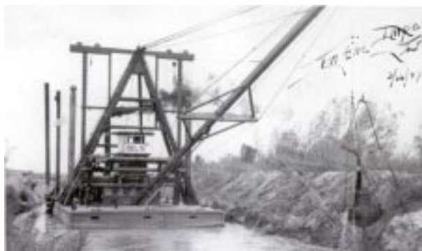
Fig. 20. Picture of the dredge Delta cutting a new canal. Courtesy of the Arizona Historical Society, Tucson.
