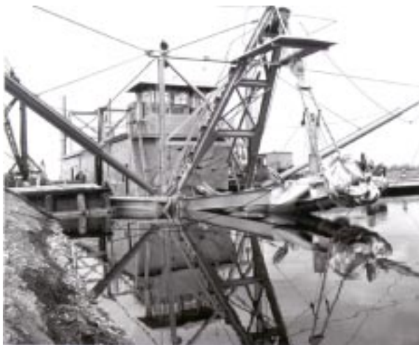
Fig. 23. The dredge Colorado straightened 30 miles of the Colorado River near Needles, California. Here the dredge is tied at Needles in 1949, P423-3000-1808A. Courtesy of the Bureau of Reclamation, Boulder City, Nevada.
