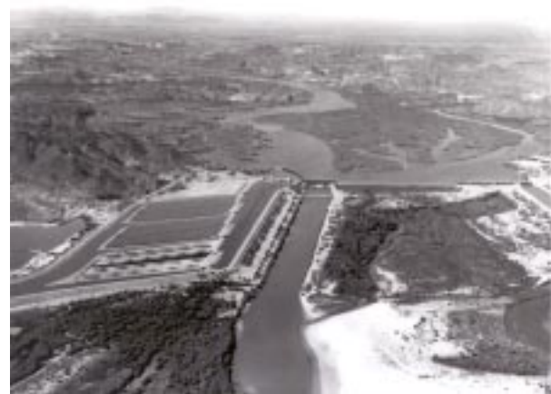
Fig. 30. Imperial Dam, P212-3000-3890-1A. Courtesy of the Bureau of Reclamation, Boulder City, Nevada.
