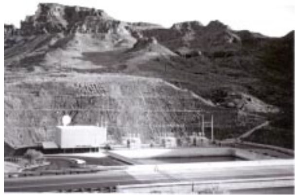
Fig. 38. Colorado River water is lifted nearly 800 feet by the Lake Havasu Pumping Plant located on Lake Havasu near the confluence of the Bill Williams River.
