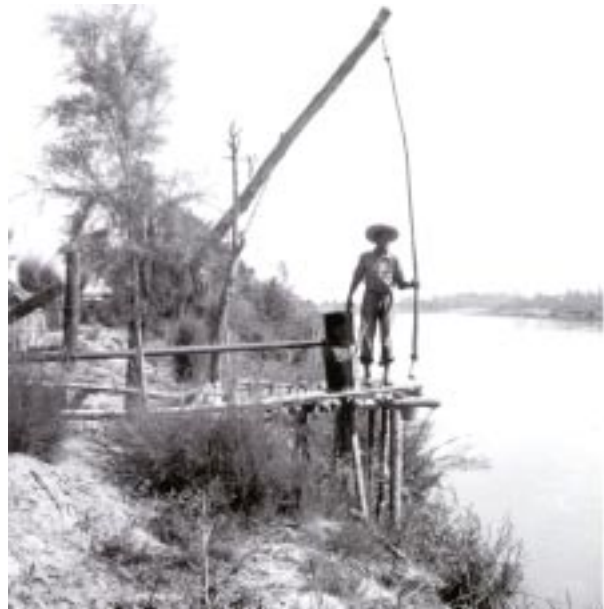
Fig. 18. Primitive water lift believed to have been located in the Colorado River delta (date unknown). Courtesy of the Bureau of Reclamation, Yuma, Arizona.
