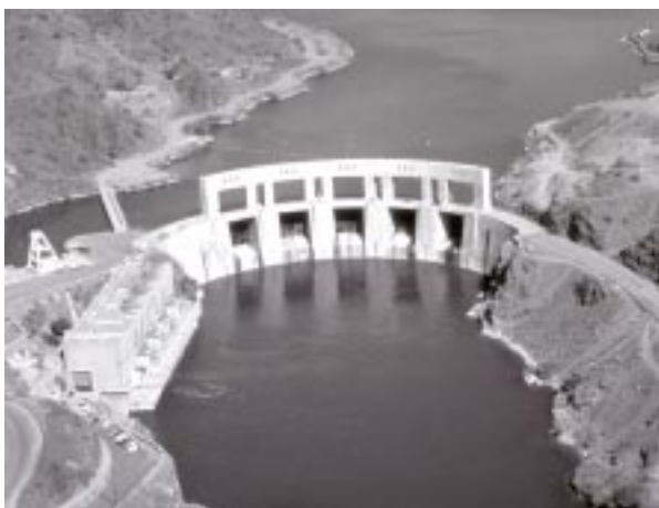
Fig. 29. Parker Dam. Courtesy of the Bureau of Reclamation, Boulder City, Nevada.
