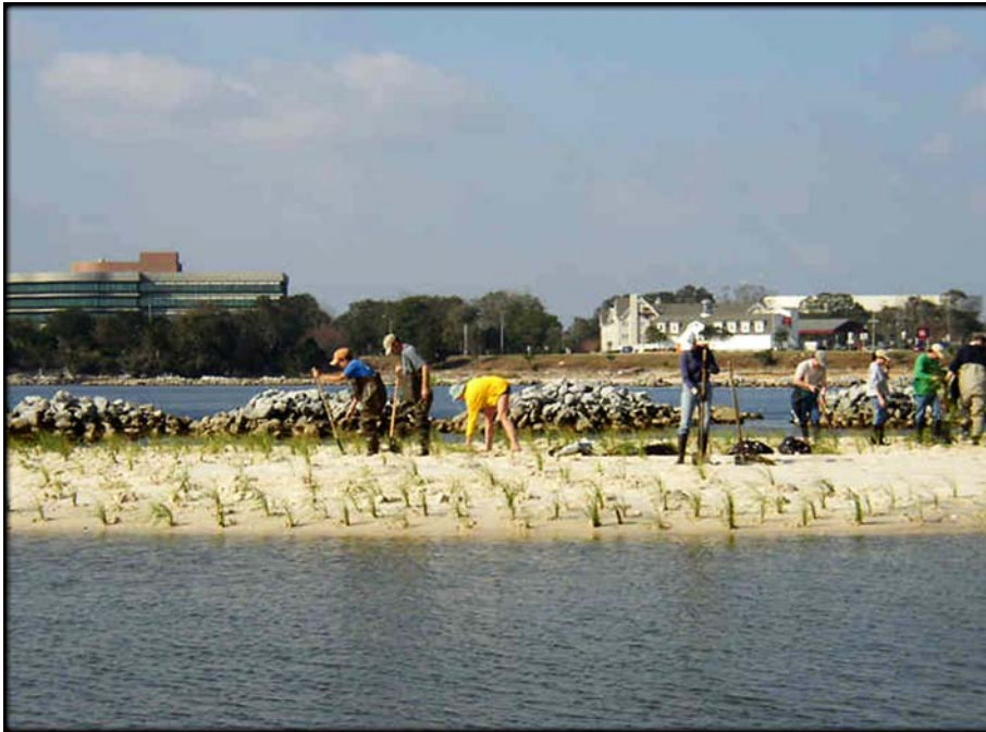
Project GreenShores — Volunteers plant saltmarsh grass behind the newly created oyster reef/breakwater.
