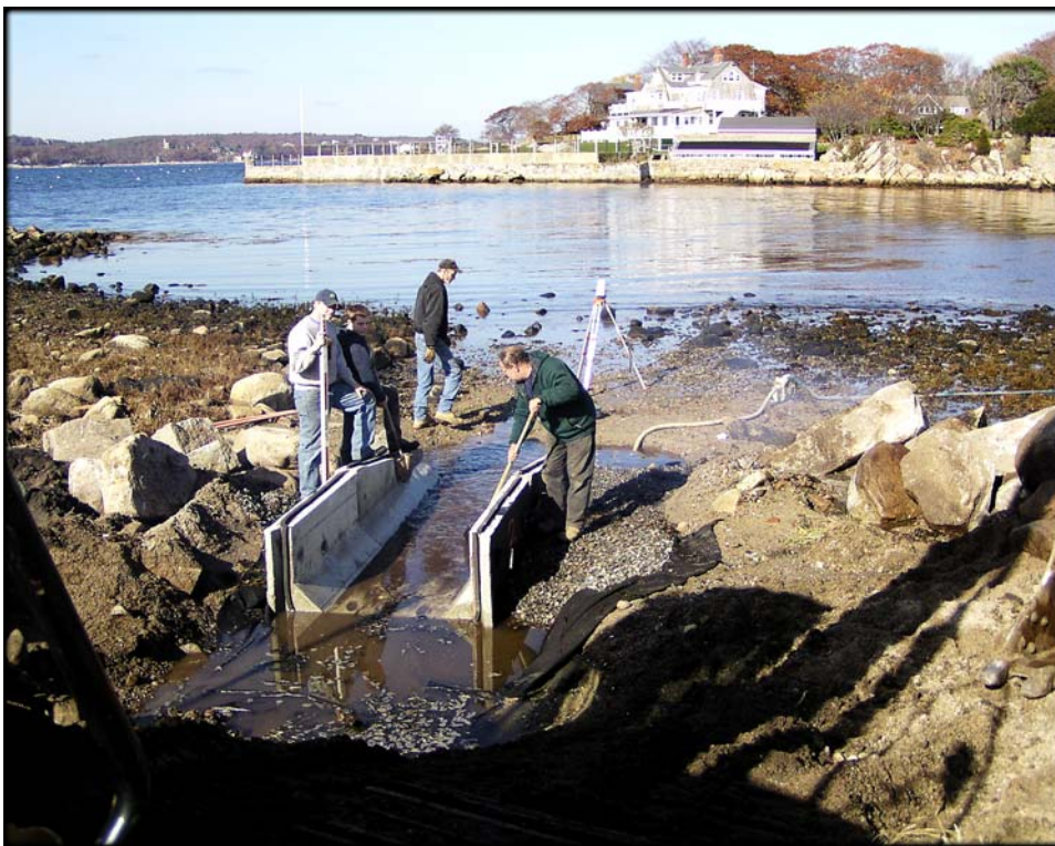
Construction of a culvert in the Eastern Point Salt Marsh.
