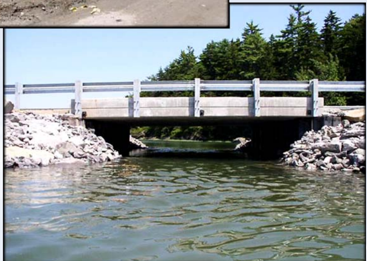
The completed bridge, which allows tidal flow restoring 45 acres of clam flats near Dingley Island, ME.
