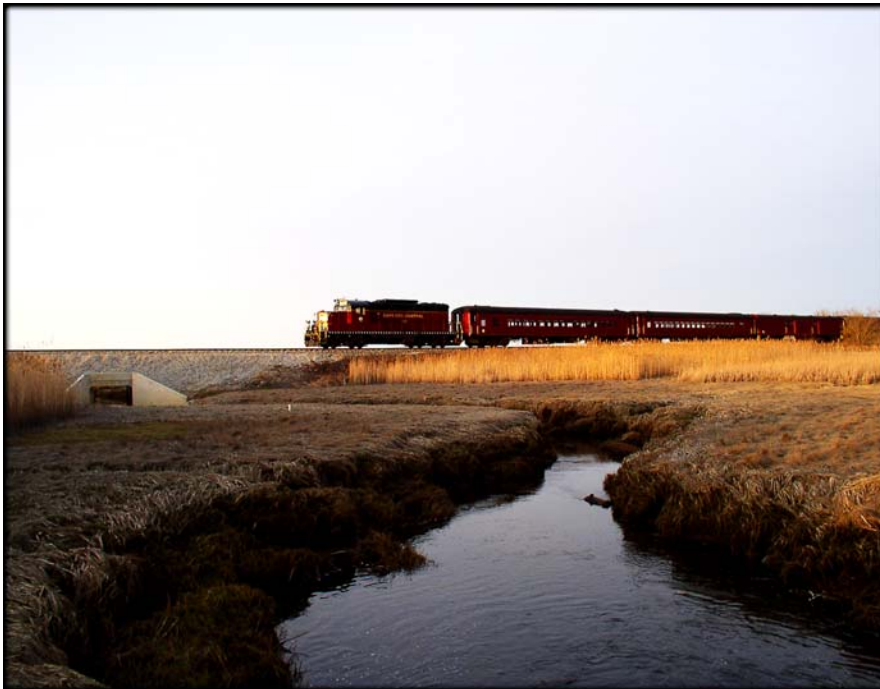
The Massachusetts Chapter of CWRP donated funds and services valued at over $90,000 to restore tidal flow under the Bay Colony Rail Line.
