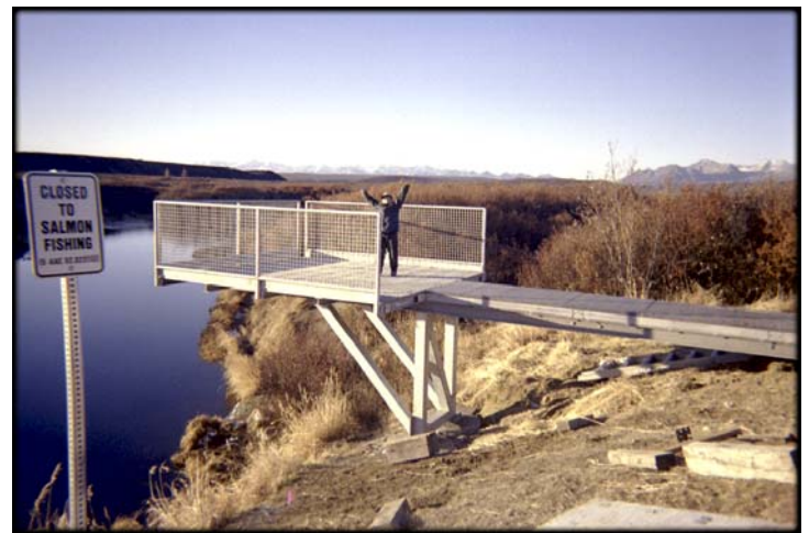
The nearly-finished observation platform.
