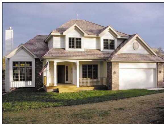
The Research Demonstration House, built on FPL grounds, is being used to monitor moisture intrusion and promote proper building practices.
