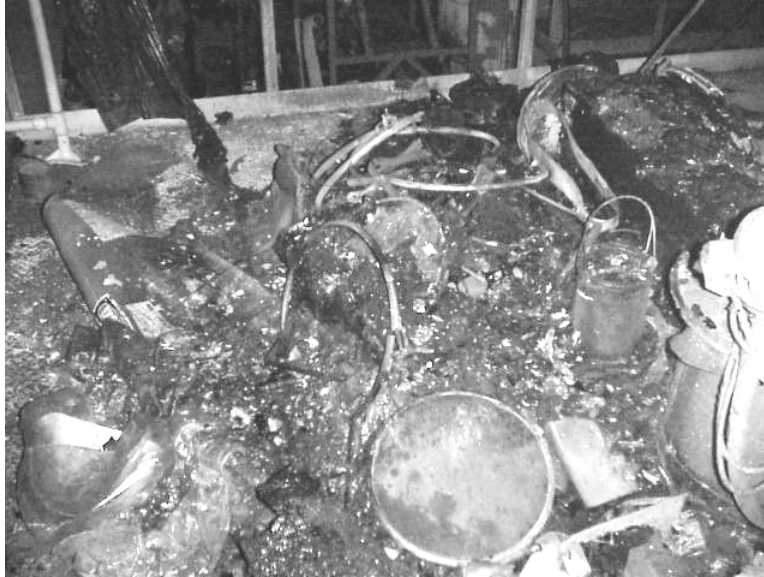
Figure 7. Remains of acid hood on mezzanine 1.
