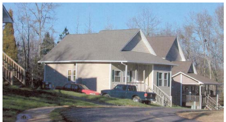
New housing at the Catawba Indian Nation, South Carolina
