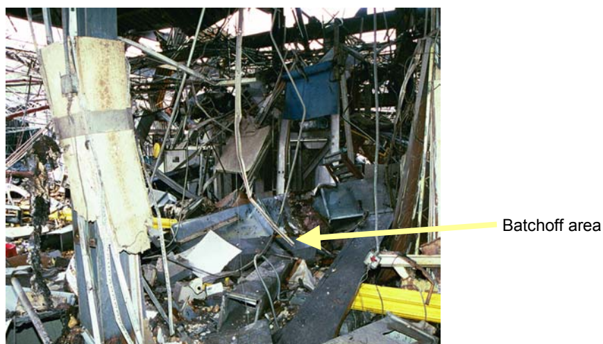
Figure 11. Extensive damage and debris near mill and batchoff machine #1.
