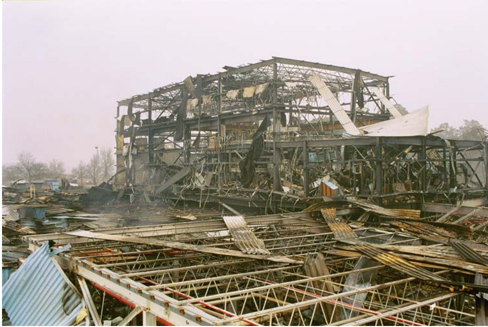
Figure 6. Roof of facility, with two-story compounding section in background.
