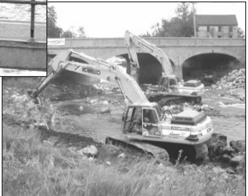
The East Machias dam was removed by a Coastal America team including Air Force Reserves working through the IRT Program.
