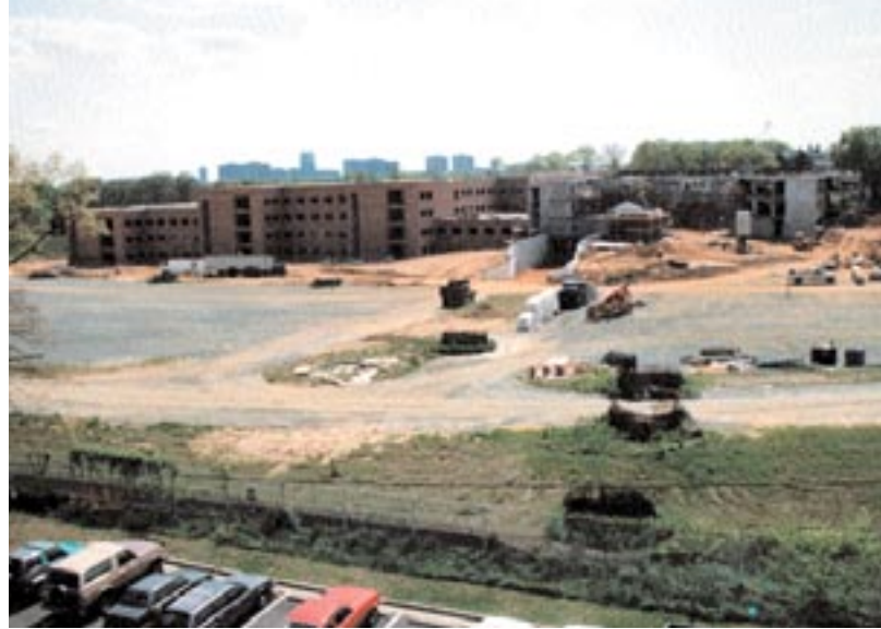
Construction progresses on the NFATC campus in April 1992.
