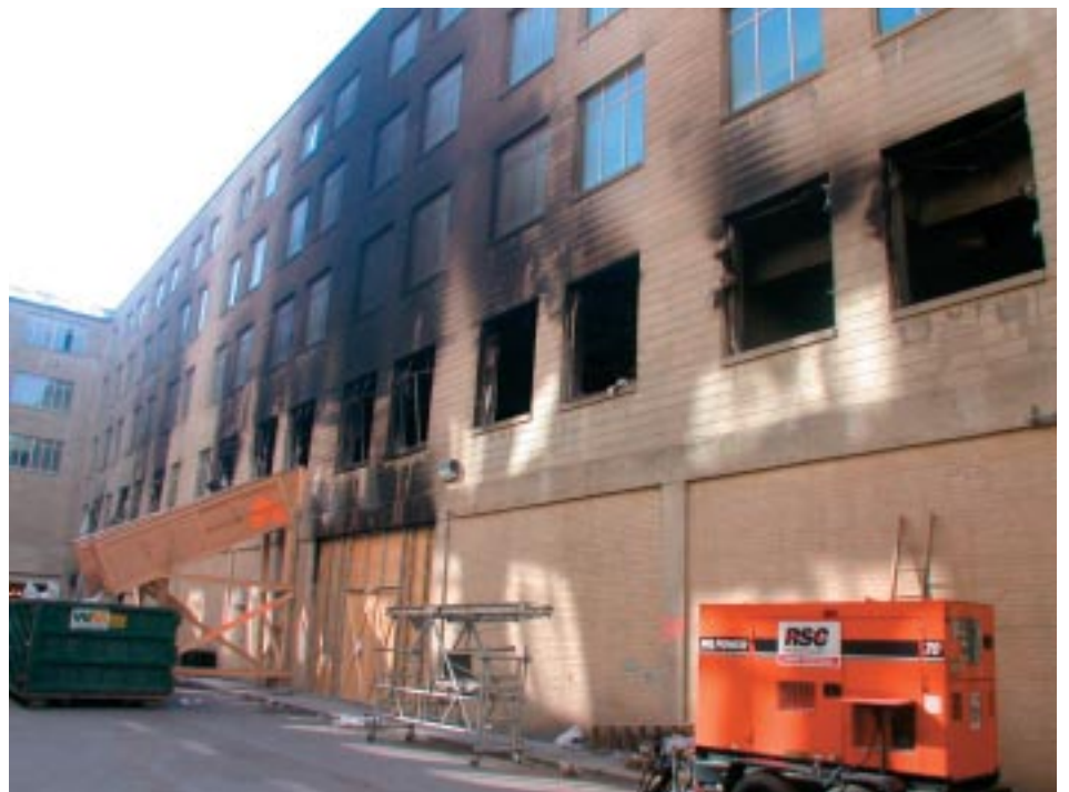
Blackened walls recall the fire's fury.
