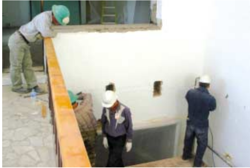
Mongolian crew works on wellness renovations.
