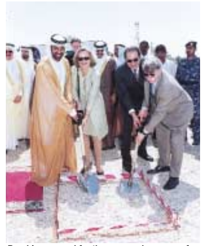
Breaking ground for the new embassy are, from left, Sheikh Khalid Al Hamed; DCM Deborah K. Jones; former Ambassador Theodore H. Kattouf; and OBO's Joseph Toussaint.
