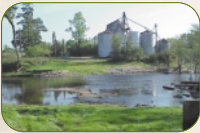
The Rains Mill Dam, before, during and after demolition; NC.
