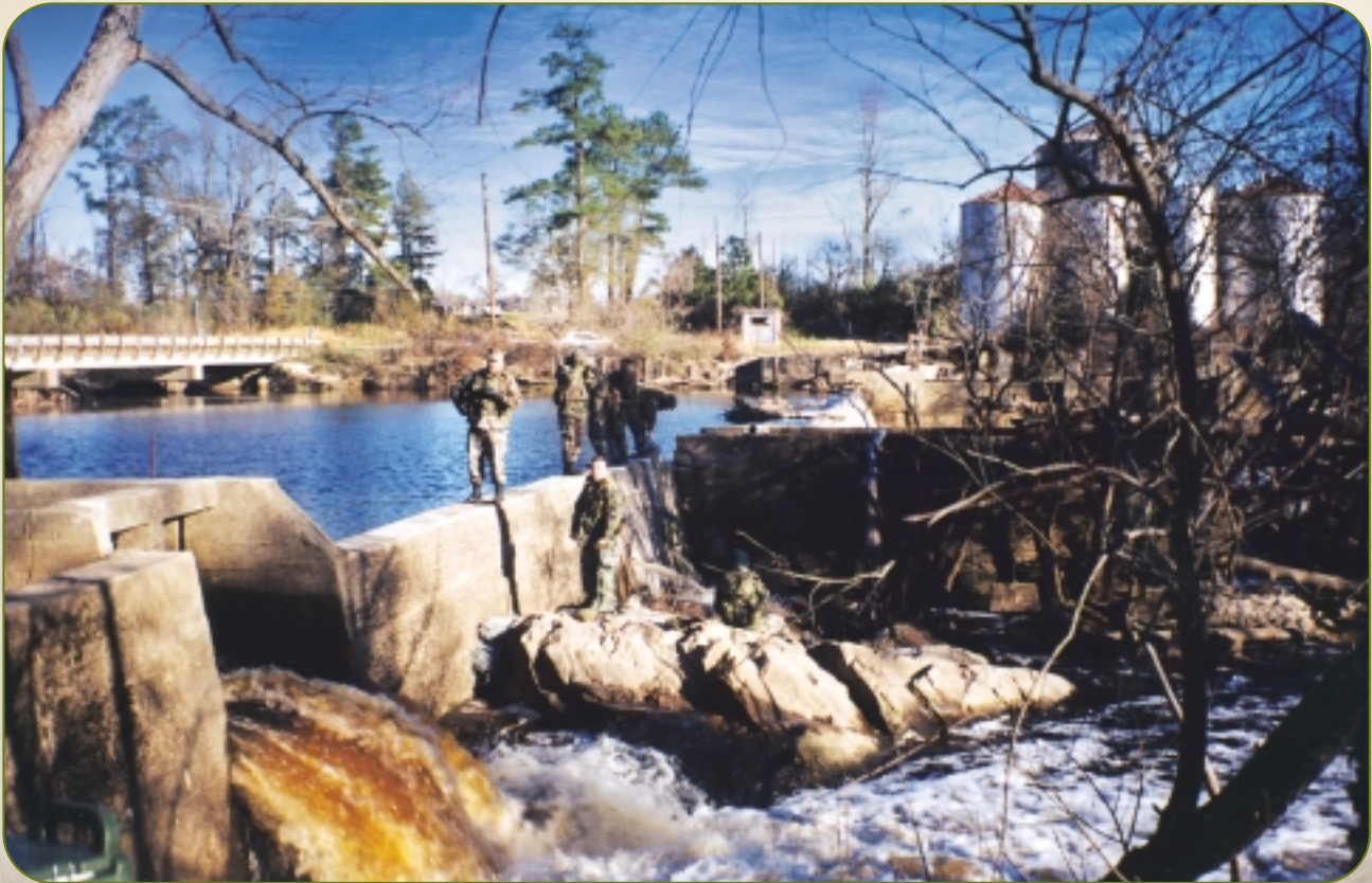
The U.S. Marines used explosives to remove the obsolete Rains Mill Dam; NC.
