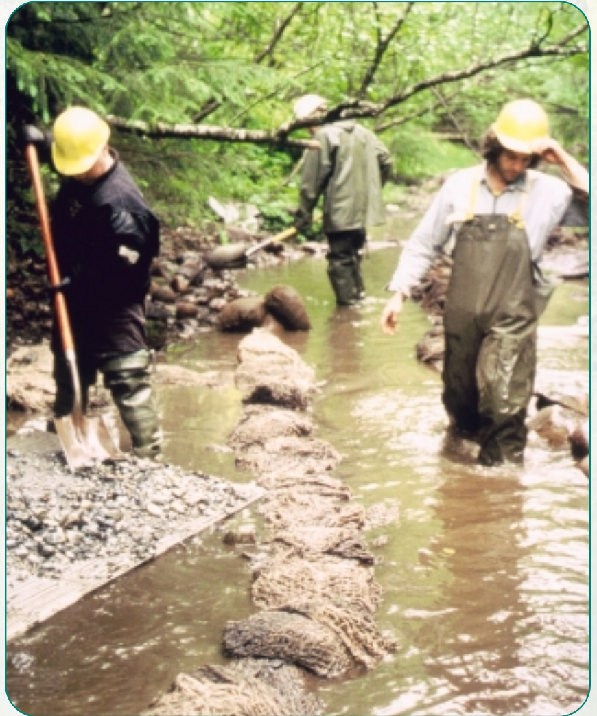
Restoration work at Duck Creek; AK
