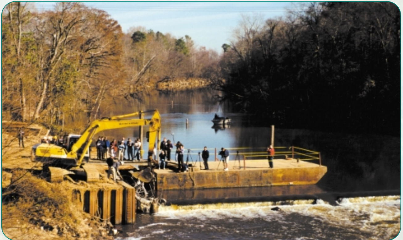
Removing the Quaker Neck Dam opened 1,000 miles of spawning habitat; NC
