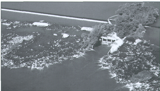
Little Falls Dam and pumping station on the Potomac River in Maryland.
