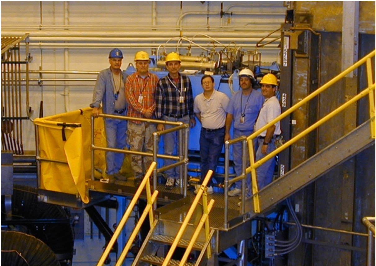
Staff responsible for the installation of the third and final long-pulse ion source on the NSTX neutral beam are (from left) Paul Ernst, Len Halvorsen, Martin Wisowaty, Mark Cropper, Kris Gilton, and Ed Bush.
