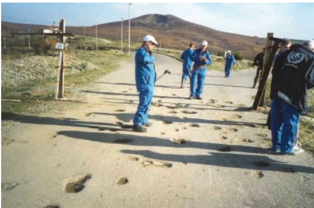
At Radoniq/Radonjic Lake the road to the dam had been hit by cluster bombs and DU penetrators.
