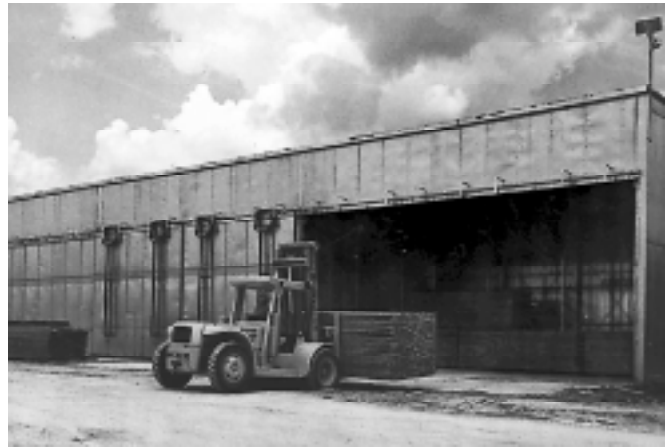
Figure 5—Typical package-loaded dry kiln.
