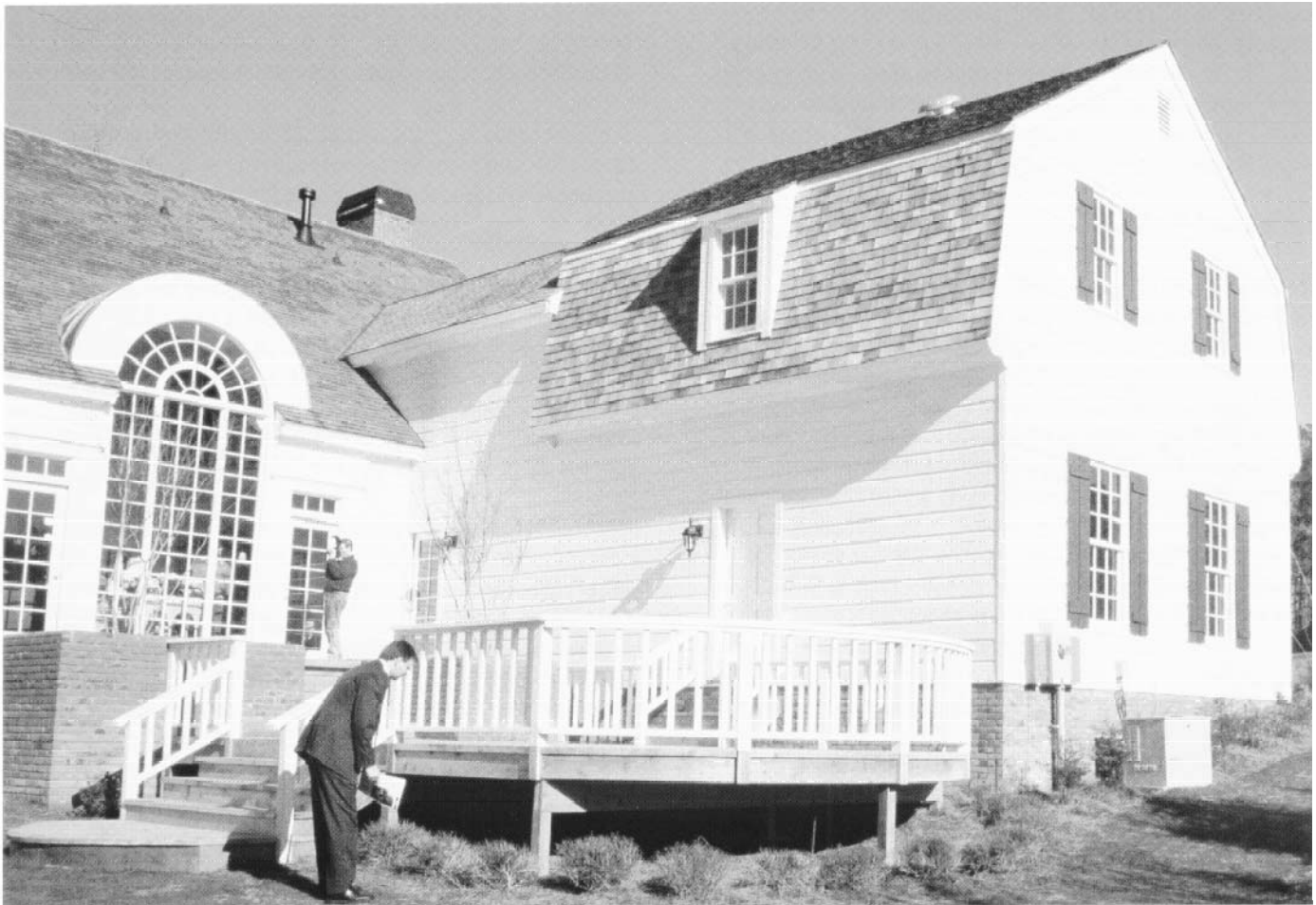
Figure 27---Commercial structure with wood shingle roof. (Photo courtesy of Southern Forest Products Association.)
