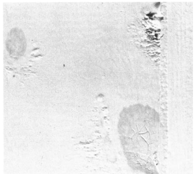
Figure 42—Brown discoloration of paint caused by resin exudation from a knot. (M84 0492-4)
