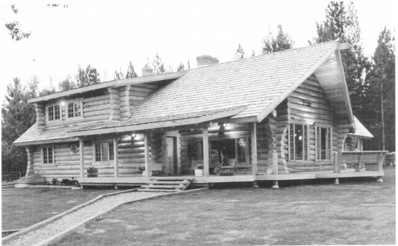
Figure 28—Log house with wood shake roof.
