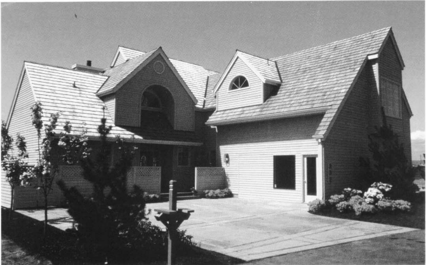
Figure 24—Modern houses finished with semitransparent penetrating oil-based stains. (Photos courtesy of Southern Forest Products Association.)
