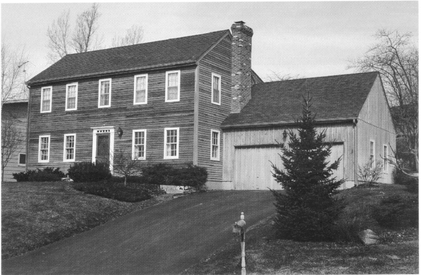
Figure 14—House with western redcedar siding that has been allowed to weather naturally.
