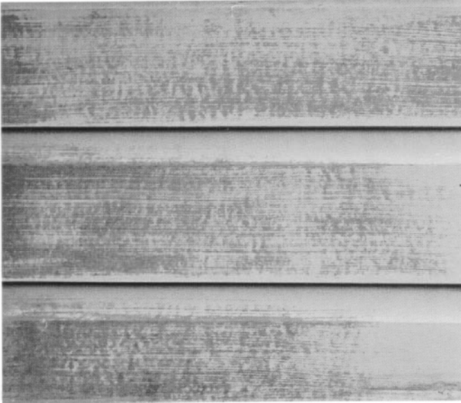
Figure 32—Mildew on paint is most common in warm, humid climates. It also occurs in shaded or protected areas.
