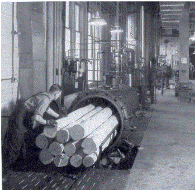
This 1934 photo shows a load of fence posts being inserted into the preservation cylinder at the Forest Products Laboratory treating facilities.
