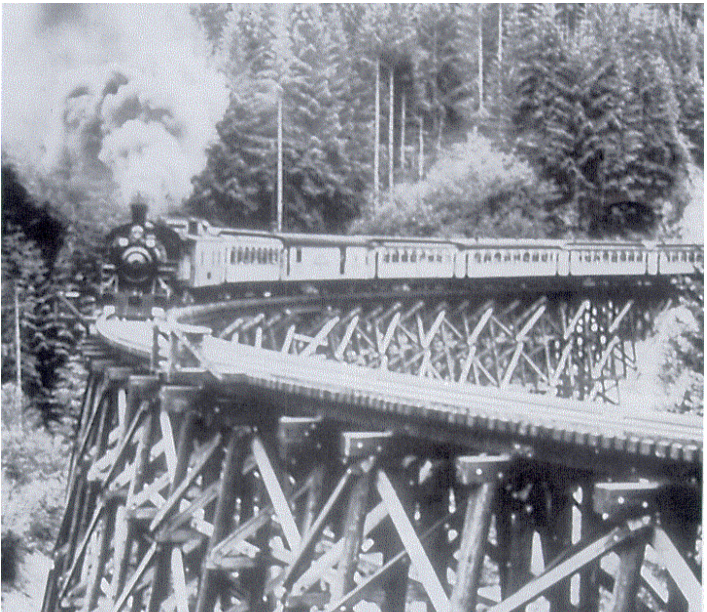
Timbers required for railroad ties and bridges put great pressure on U.S. forest resources. Railroad ties were untreated with preservative until after 1910, which resulted in replacement of ties on 50,000 miles of track annually. Some of the Forest Products Laboratory's earliest research developed effective preservatives, which reduced the replacement rate for ties and decreased harvest pressure on forests. Shown here—A wood railroad trestle.
