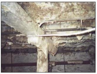
Rotten rafters caused by decay. (Photo used with permission from KBA Engineering.)
