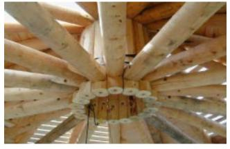
decay organisms. The *roof trusses* are untreated ponderosa pine. Critical to using roundwood timbers are the connections.
