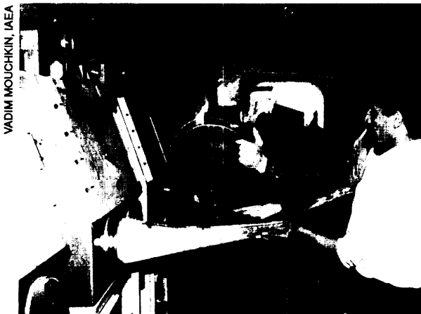
Under IAEA supervision in October 1991, Iraqi workers pour concrete into glove boxes at Al Tuwaitha to prevent their future use. Glove boxes are used to protect workers from radioactive materials such as plutonium.
