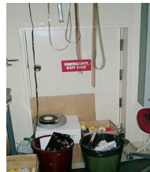
Emergency Exit from Projection Room Blocked
