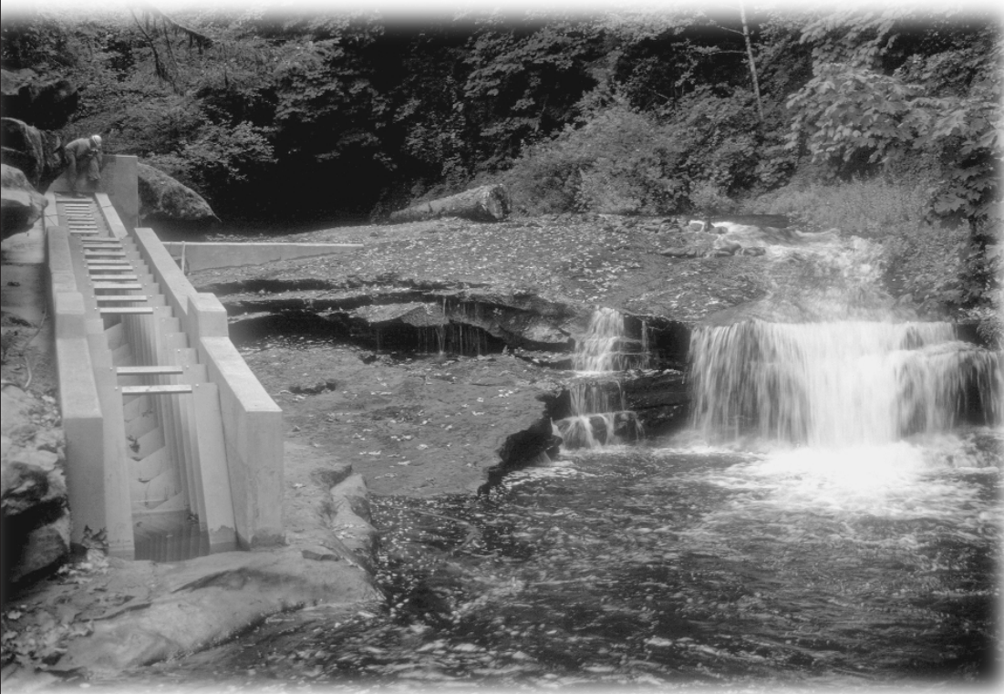
A fish ladder on Lake Creek in Oregon restores migration routes for native fish. (photo by D. Huntington)
