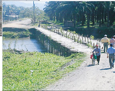
Temporary bridge erected after hurricane
