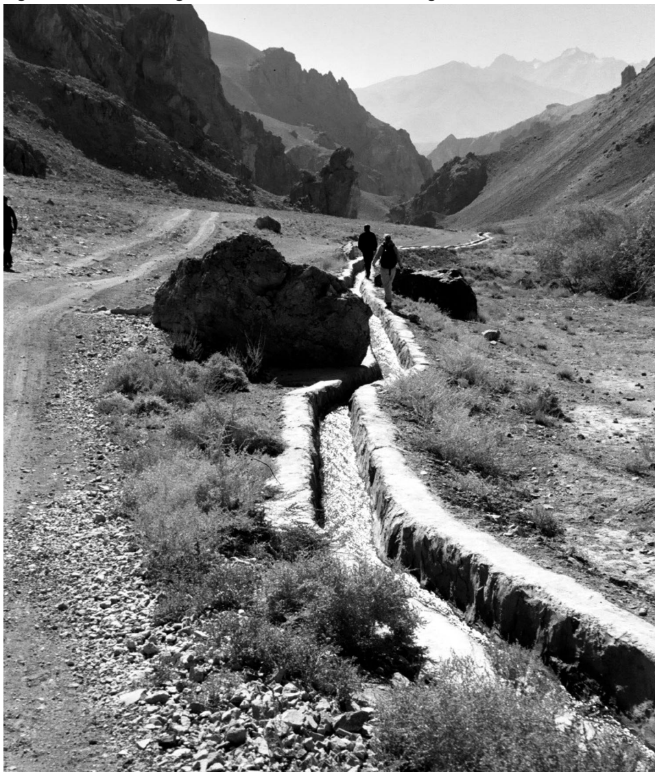
Figure 8: Fatmasti Irrigation Canal outside Bamian, Afghanistan
