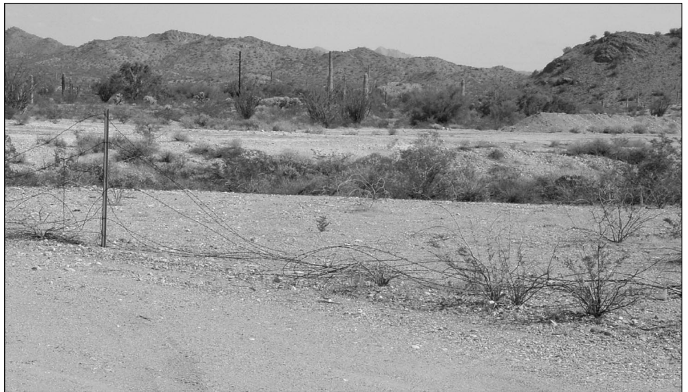
Figure 7: International Border Fence on Federal Land in Arizona, Presumed Damaged by Illegal Aliens or Smugglers
