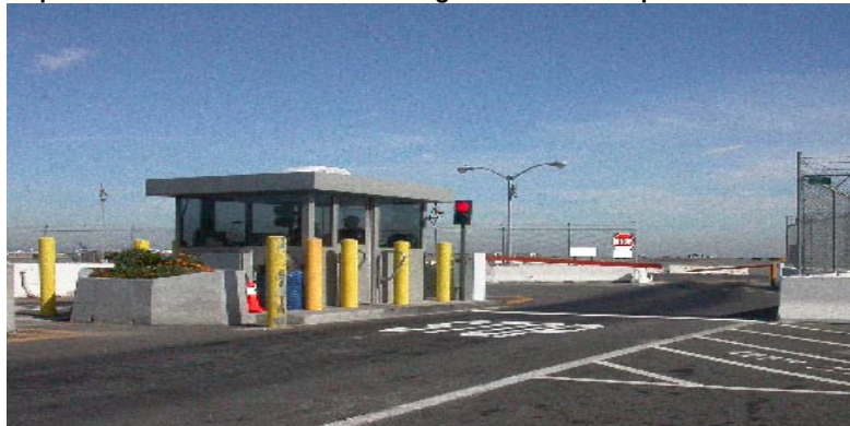
Airport Perimeter Access Gate at a Large Commercial Airport
