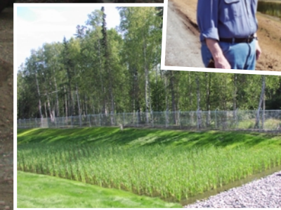
Construction of the Talkeetna sewage treatment project was completed in the summer of 2003. USDA funding amounted $1.3 million.
