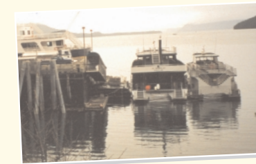
ALLEN MARINE TOURS Docking facilities for Allen Marine Tours in Ketchikan, financed through a B&I loan guarantee.
