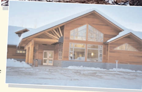
Begun in May 2003, construction of the new Sunshine Clinic was completed in January, 2004. In addition to providing health care services, the clinic also provides upper Susitna Valley with behavioral health care, and dental care. The clinic has a staff of 35, and is one of the area's largest employers.
