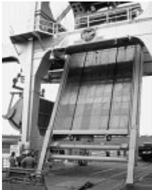
Extended-length screens, like this one at McNary Dam, guide more fish away from turbine intakes.
