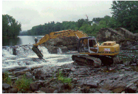
Removing a dam, to restore fish passage and wetlands
