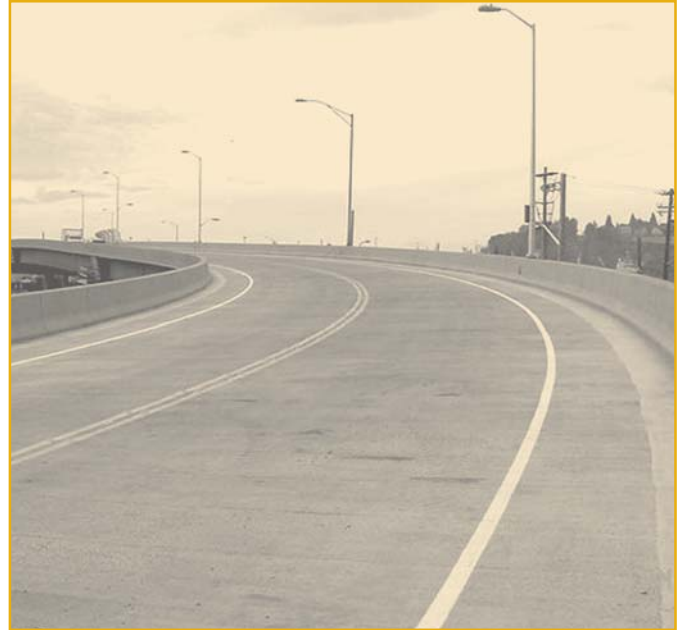
Picture of the "flyover" road (two-way access ramp) built above railroad tracks near the marine terminals.
