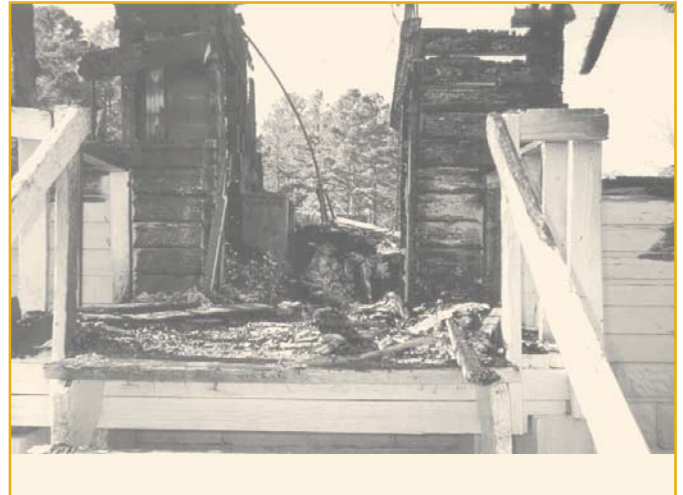
Lack of written documentation (for example, proof of fire insurance) increases the risk that RLF funds are not being administered in accordance with EDA regulations, placing federal funds at risk.
