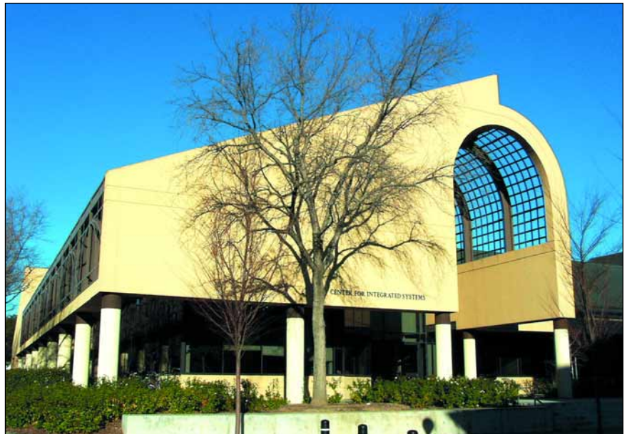
SNF is housed in the Paul Allen Center for Integrated Systems (CIS) building on the Stanford campus.
