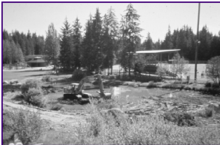
Marsh at Duck Creek, Alaska, during construction.
