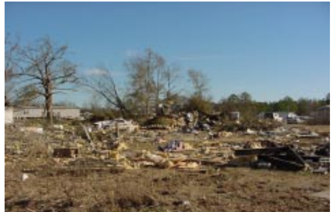
A view of the devastation at the Bear Creek Mobile Home Park.
