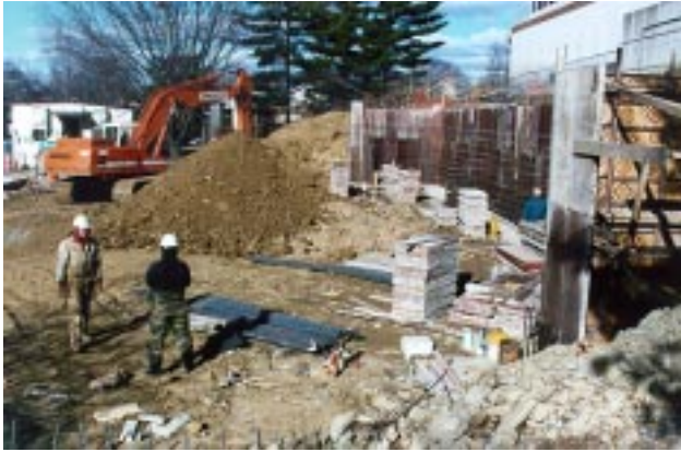
Construction is proceeding at the Cincinnati VAMC Fisher House site.
