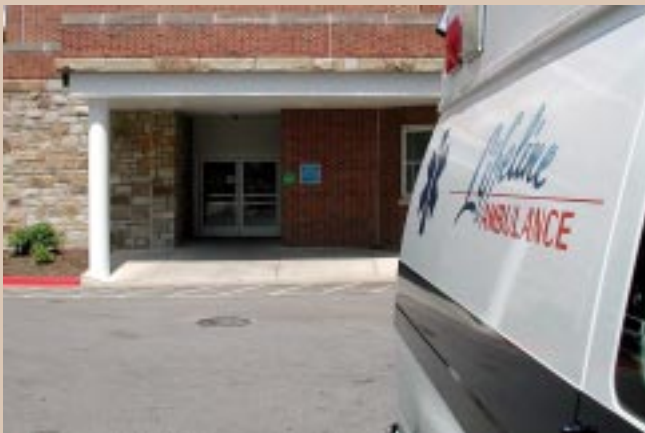
The entrance to Salem VAMC's new ER, which is equipped with a biohazard decontamination shower.
