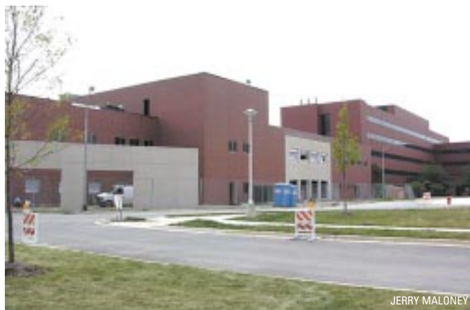
The new 34-bed blind rehabilitation center now under construction at the Hines VA Hospital is expected to be completed in late fall.
