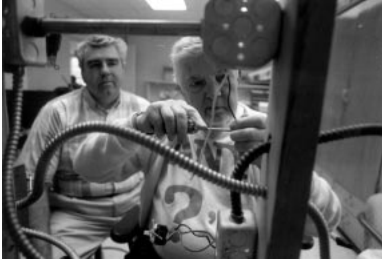
Manual Skills class at Hines VA Hospital includes home mechanics. Dieter Werner (left) assists Joe Hagerty on a wiring project.
