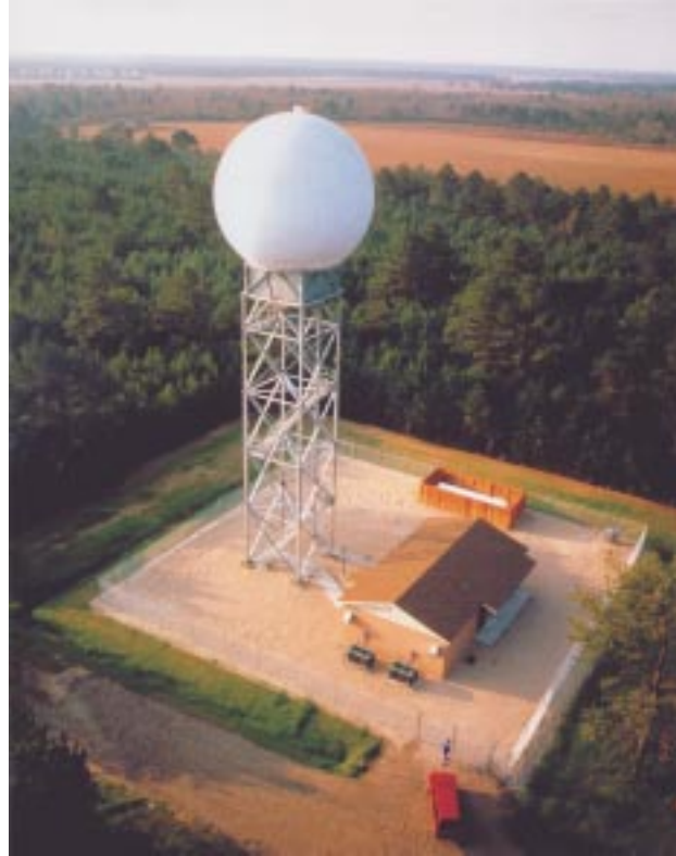
The FAA has installed Terminal Doppler Weather Radar at high-activity airports to detect weather hazards for departing and landing aircraft. Photo courtesy FAA.
