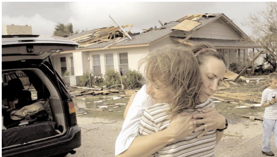
Figure 1-2. Hurricane Claudette came ashore in Texas on July 15, 2003, peeling off roofs of homes such as this one in Palacios, Texas, knocking out power, and flooding low-lying areas. (AP Wide World Photos)
