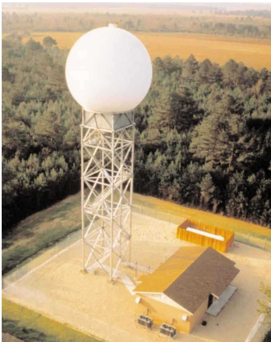
Figure 3-DOT-2. FAA Terminal Doppler Weather Radars provide supplementary wind and precipitation conditions for airport approach and departure.
