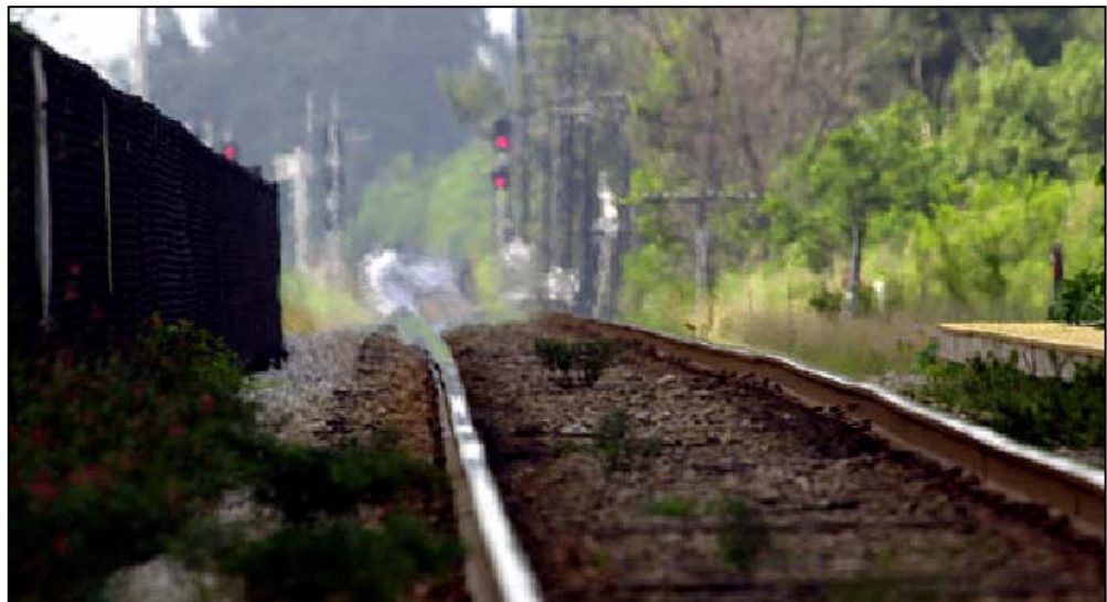
Hot air rising from a rail bed near Hollywood, Florida, gives track the appearance of being distorted. Rapid temperature changes, particularly the first of a season, can buckle rails and cause accidents. Copyright AP Wide World Photos.
