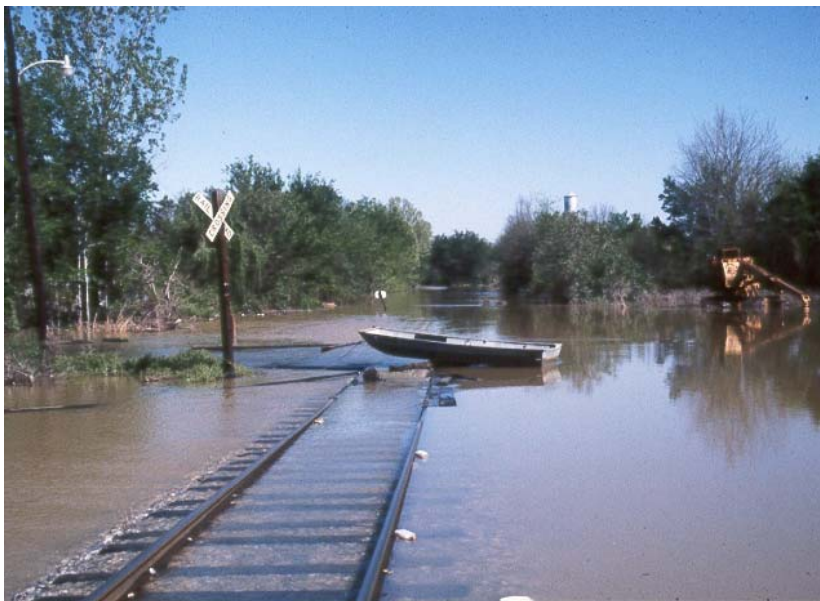
After the storm surge and heavy rain from a hurricane, obstacles lie across a flooded section of track in Alabama.
